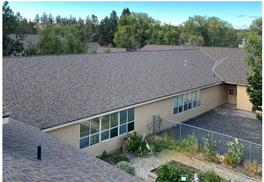
A new roof for Tumalo Community School
