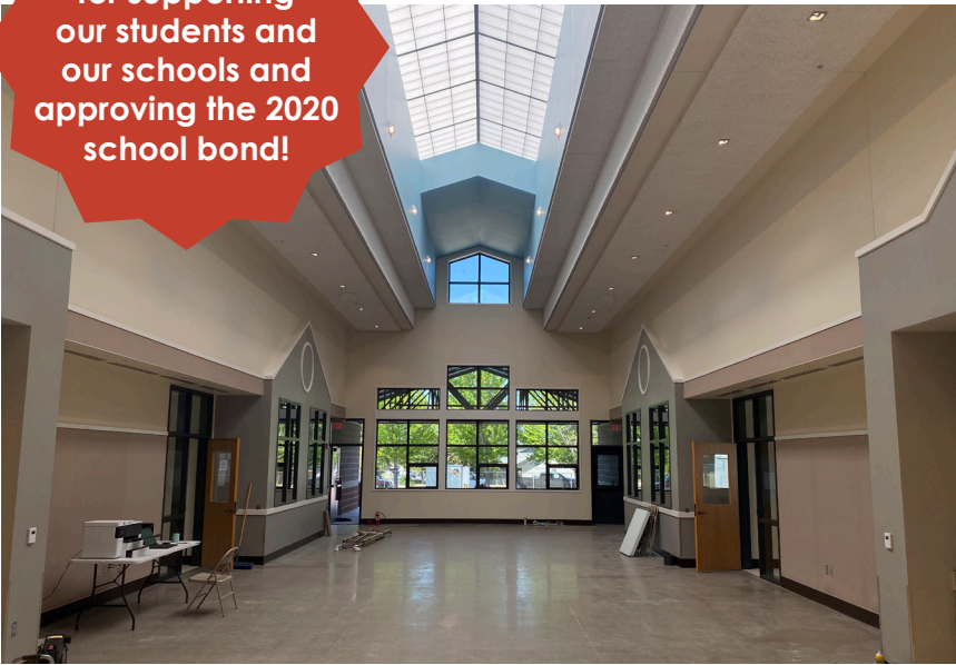
New classroom wing at Vern Patrick Elementary School
